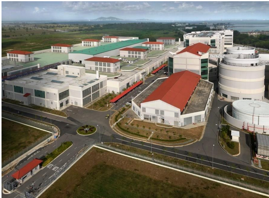
Aerial view of the Changi Water Reclamation Plant Credit: PUB, Singapore's National Water Agency
