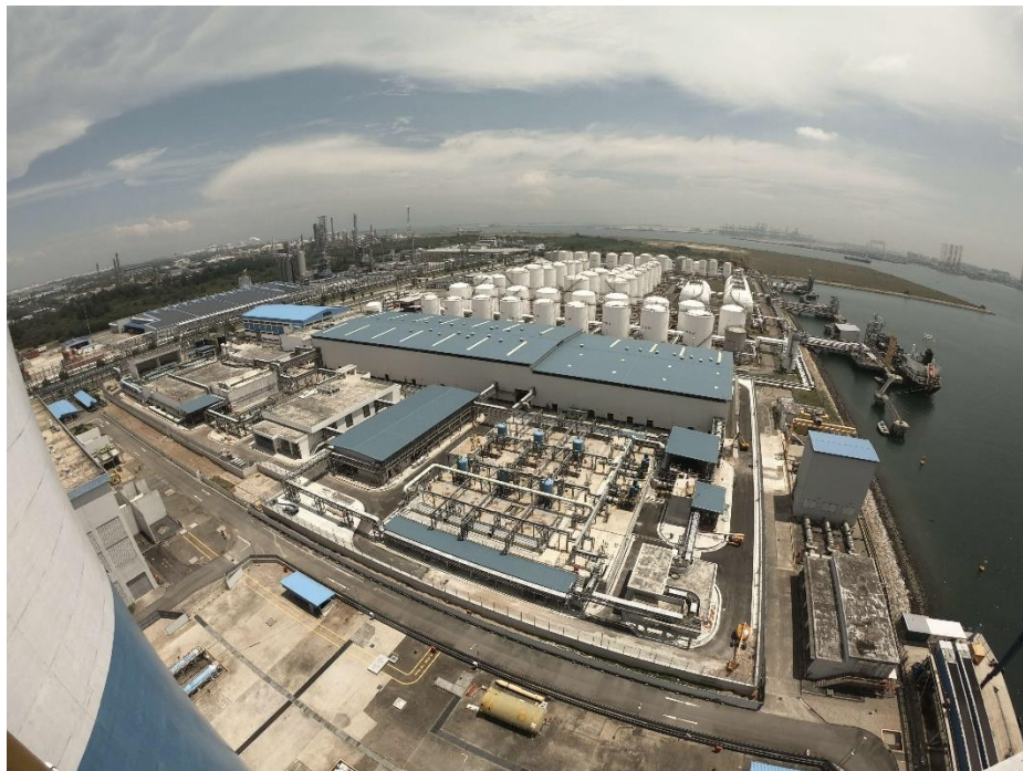
Aerial view of the Jurong Island Desalination Plant Credit: Tuas Power
